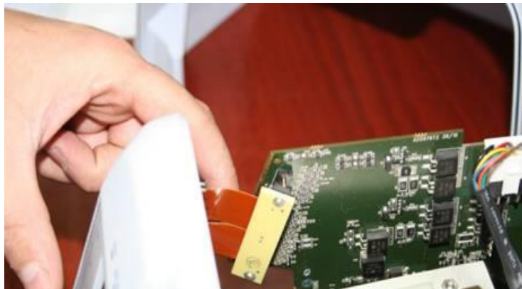
Figure 20 – Flat Flex Cable going to P16
